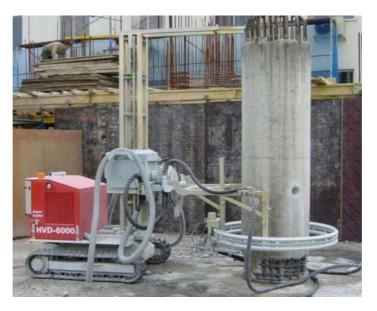
Typical Hydro-demolition Pile Breaker
